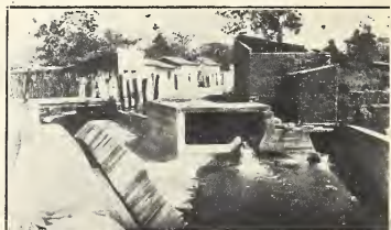
FIG. 7. The junction of two side drains with a main drain in Maracay in the Republic of Venezuela is shown in this cut. A central channel has been cut in the main drain to increase the velocity of the residual flow.
